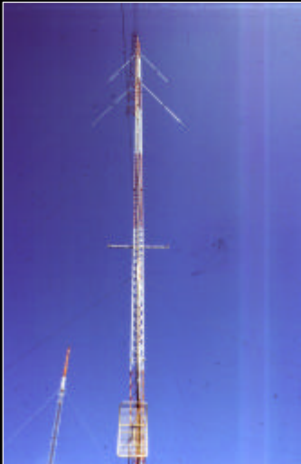
The tower for KPDJ-FM at Kneeland Mountain, elevation 2680 ft. Ten bay CP antenna atop a 200 ft. tower.
