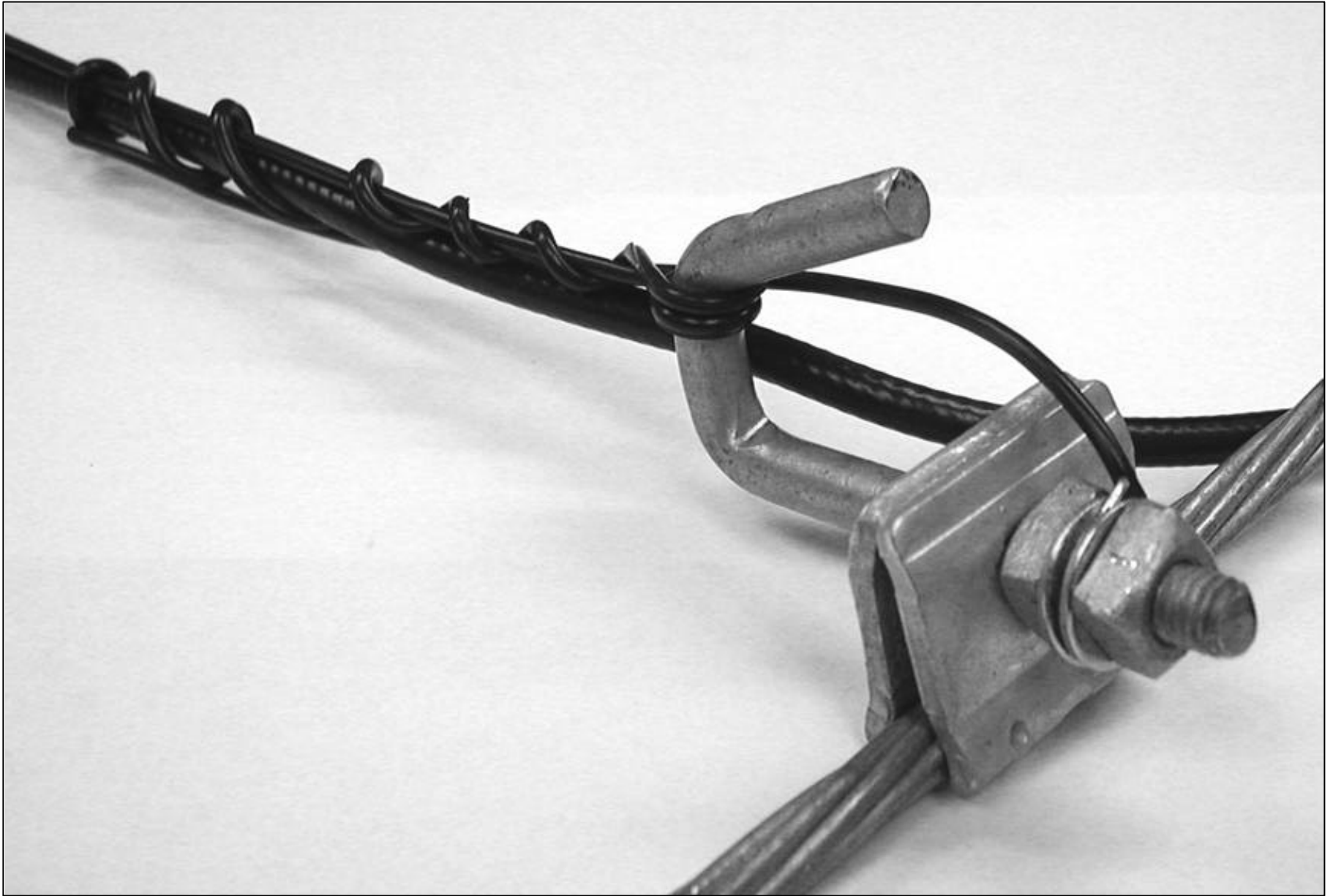
Figure 1. Strand-Grounded Span Clamp
